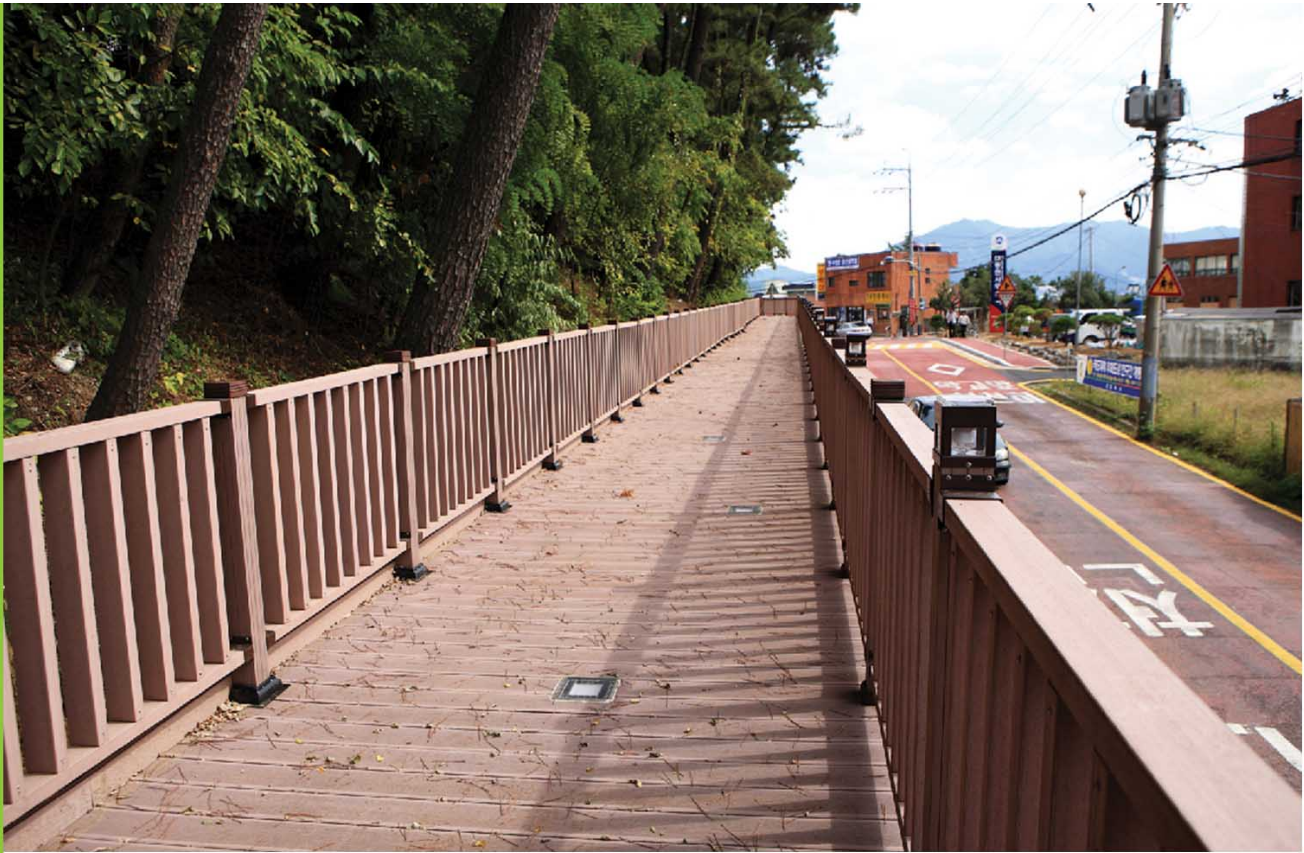
Building a pedestrian path near road
